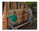
We notched a trim piece to go around the 2x4's that framed in the window openings. This piece was beveled to drain moisture like a window sill.
